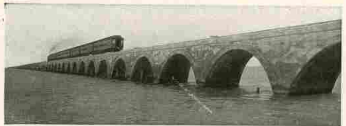
Long Key Viaduct An Important Link in the Over-Sea Railroad
